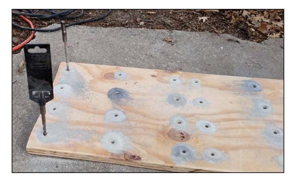
When creating a repeatable pattern of domes or a path of travel for bars the wooden template should be moved up half a section at a time and the anchor points should be set before drilling the next set of holes.
