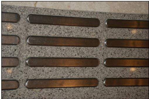
M. Do not allow foot traffic on installed Domes/Bars until the adhesive has cured sufficiently. Curing time is weather dependent (average cure time at 75° F is 30 minutes).
